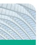
Transparent polycarbonate sheet allows natural light to enter buildings. Because polycarbonate is very light weight compared to other building material, less energy is needed for transport and installation, and boldly designed and large sizes are possible. As a highly break- and shatter-resistant material with practical inflammability polycarbonate filfills the critical fire safety standards and regulations regarding safety of buildings.
